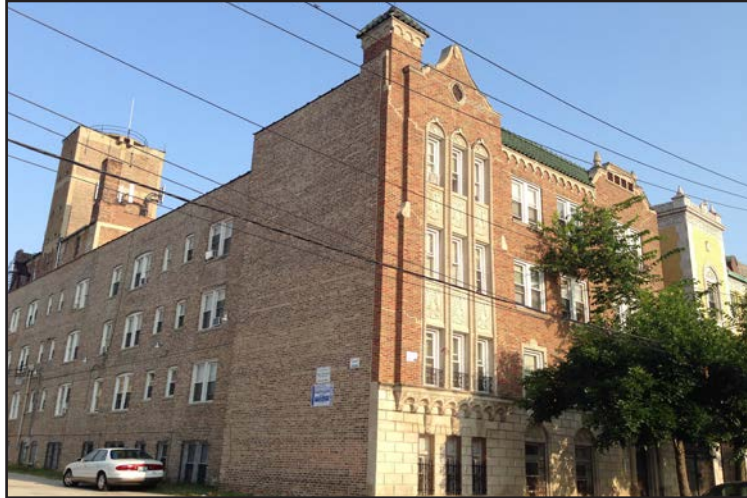
6 10 SOUTH MASON AVENUE Chicago, IL 60644
