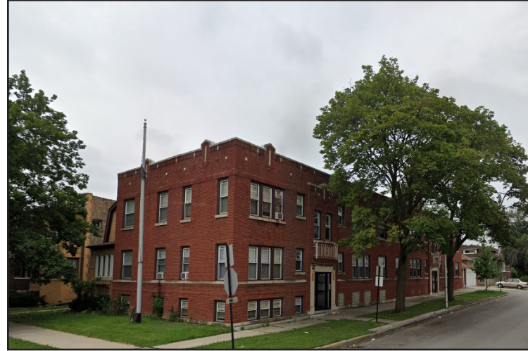
3 5901 WEST FILLMORE STREET Chicago, IL 60644
